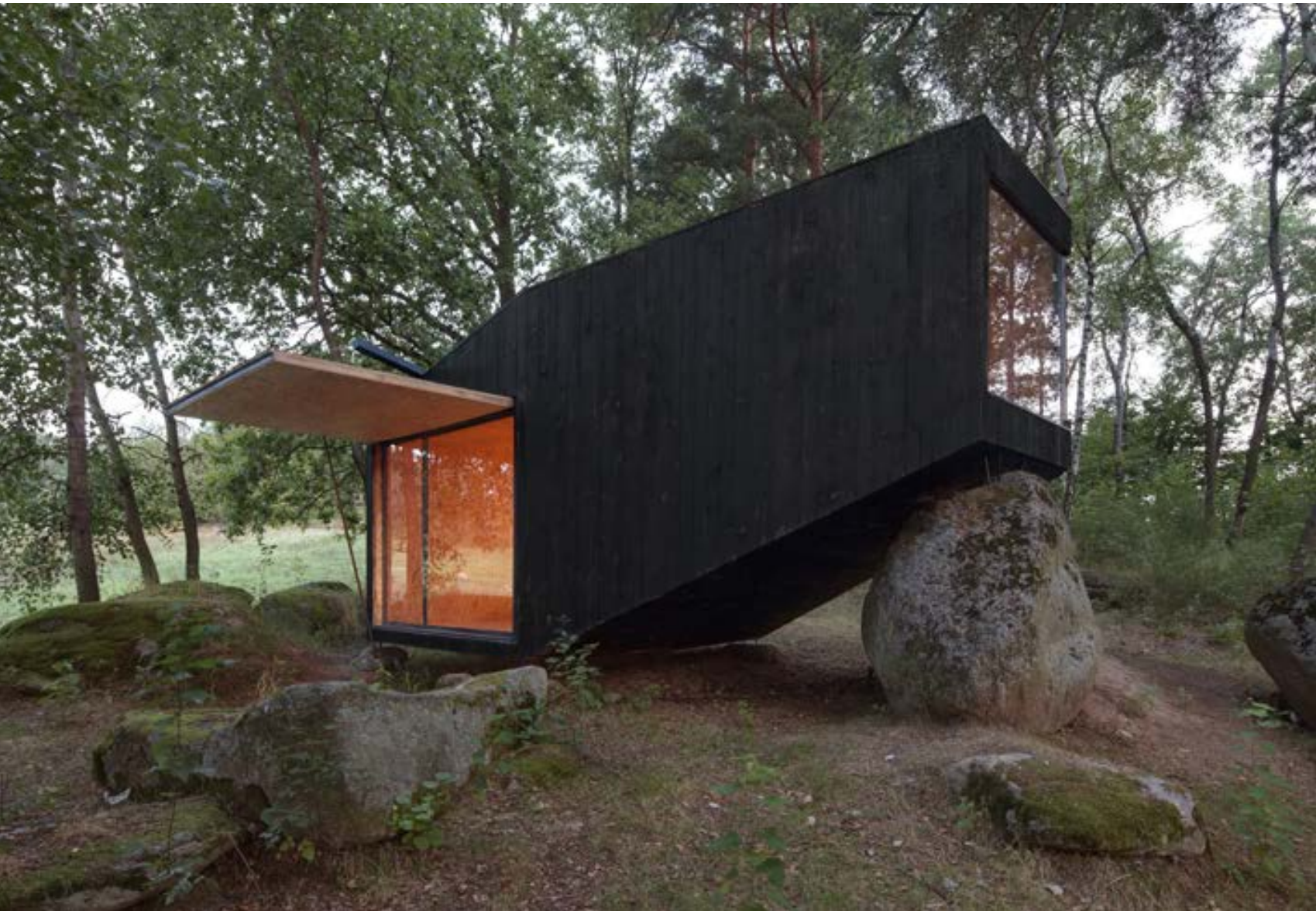
↑↓ Directly engaging with its natural surroundings, the structure uses a boulder as a plinth.
