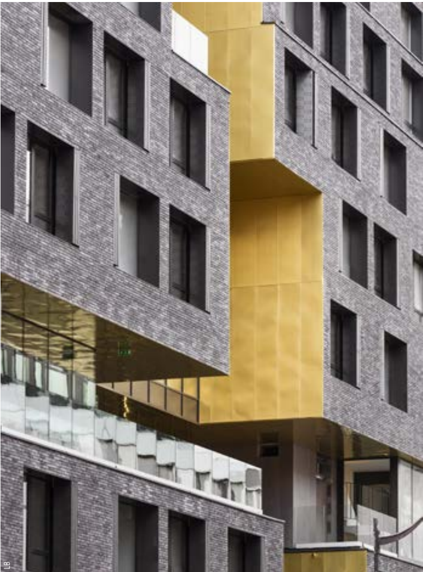
↑↓ The eye-catching block has a skin of anthracite brick accented with gleaming copper.
