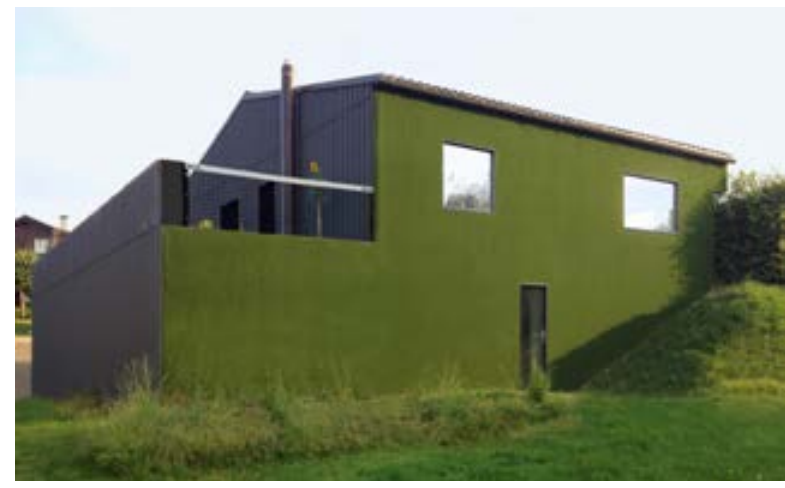
↑ Rear facade covered in artificial turf ↓ View of the facade facing the street
